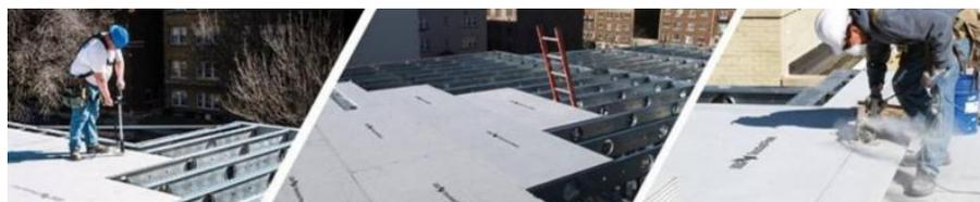
USG Structural Panels are reinforced concrete panels designed for assemblies and non-combustible construction. They install like wood sheathing and are:
